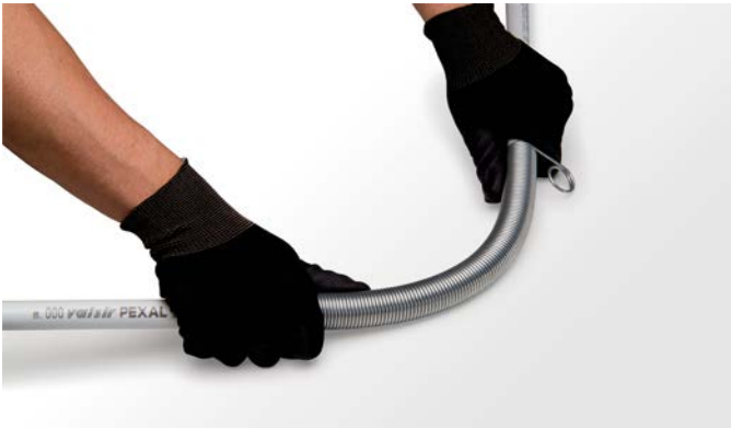
Figure 8.34 Bending with external spring.
