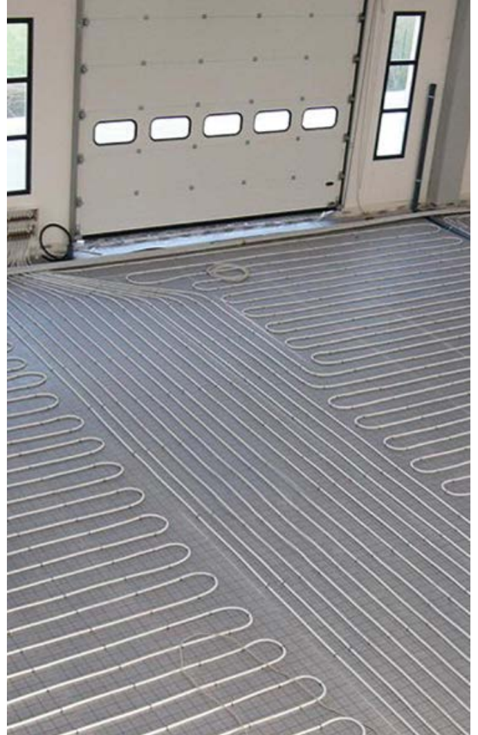
Warehouse - Sondrio (Italy)
